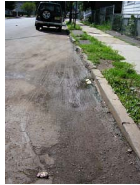
Road conditions along Howard St. [facing Georges Rd.] 98
