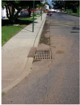
Pine St. intersection with Nichol Ave. looking towards Georges Rd.
