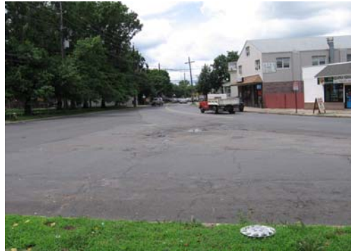
Problem intersection [Powers St. to the right, Jones Ave. to the left]
