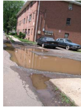
Parking lot of apartments [showing poor drainage]
