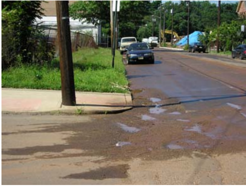
Poor road conditions and drainage at intersection of N. Ward and Commercial Ave. 91
