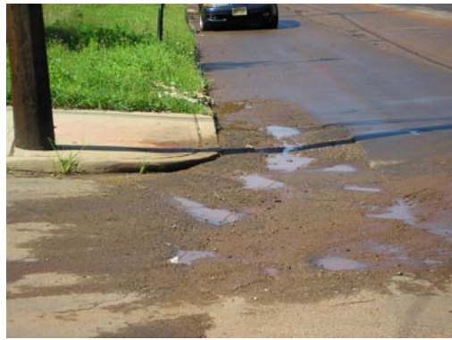
Close up of road conditions 92
