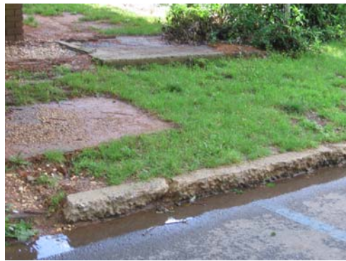
Sidewalk ending right after apartments
