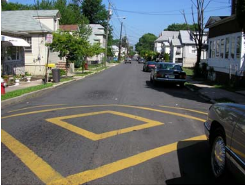
Speed hump on South Ward St. 86
