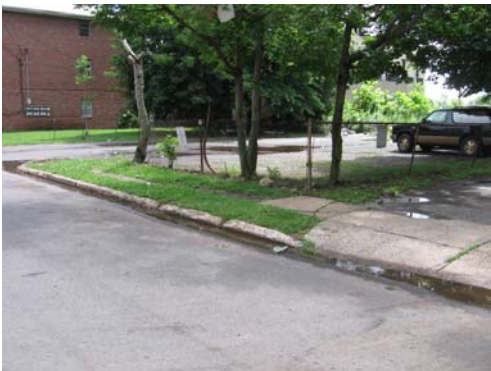
Reservoir Ave, near dead end [illustrating poor drainage system and a desire path]
