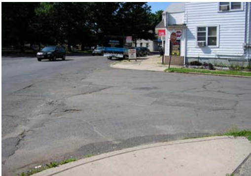
Looking across Powers St. at intersection with Georges Rd. [illustrating lack of a sidewalk]
