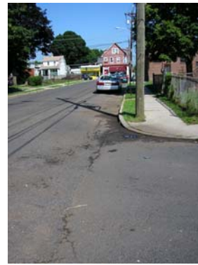
Corner of So. Talmadge and Kempton Ave. looking towards Georges Rd.
