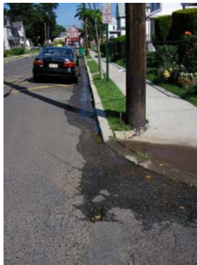
Corner of So. Talmadge and Nichol Ave. looking towards Georges Rd.
