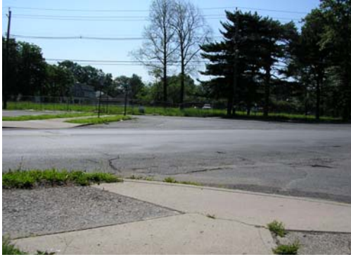
Problem intersection looking across Georges from left corner of Powers
