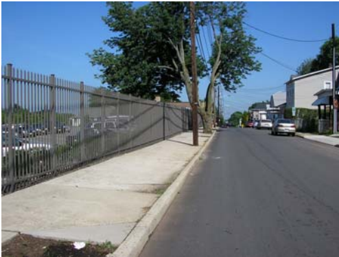
South Ward St. sidewalk bordering Bristol Myers property 88
