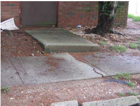
Condition of sidewalk outside apartments on Reservoir Ave.
