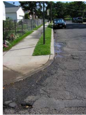
Corner of So. Talmadge and Nichol Ave. [flooding problems and poor drainage]
