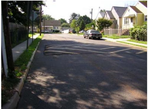
Speed hump on So. Talmadge near Mason Ave. (looking towards Larch Ave.) 63
