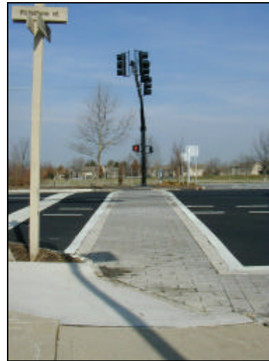
Figure 3: After – Signal, Textured Crosswalk
