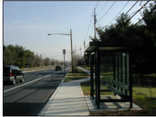
Figure 5: After – Bus Shelter
