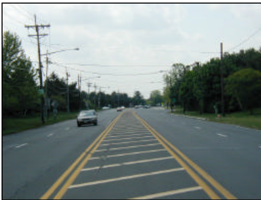
Figure 7: Before - Flush Median
