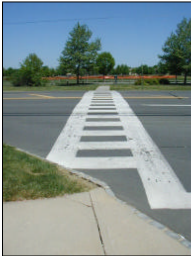
Figure 2: Before – No Signal, Striped Crosswalk
