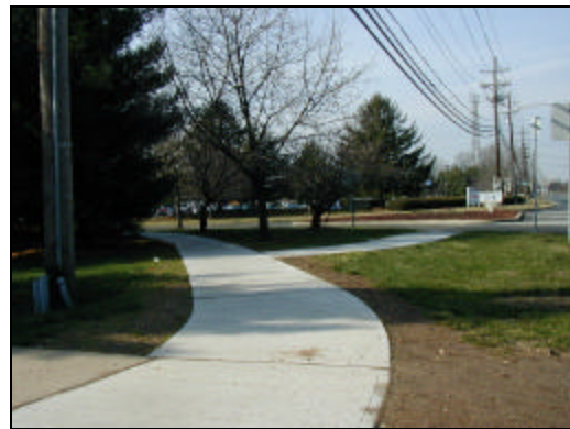
Figure 9: After – Concrete Walk
