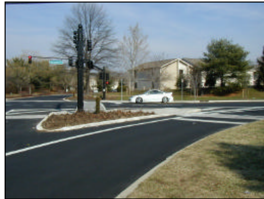
Figure 10: After – Signal, Larger Island, Crosswalk and Channelization
