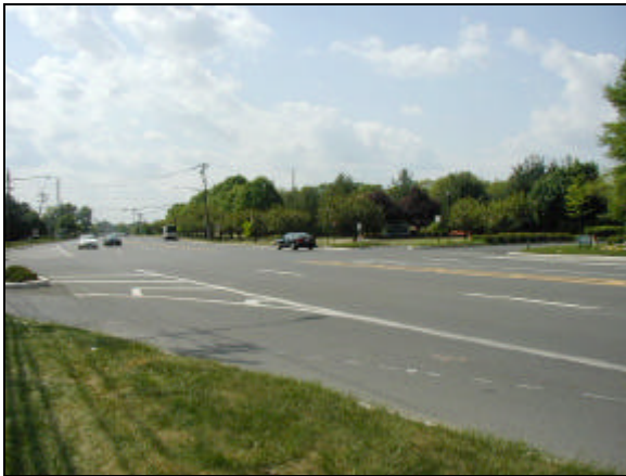
Figure 3: May 2001 at Hunters Glen-Deer Creek Intersection
