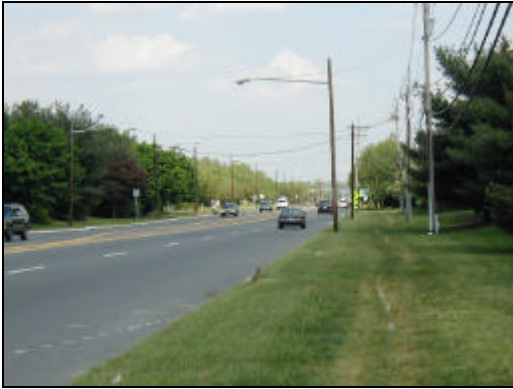
Figure 4: Before – No Bus Shelter
