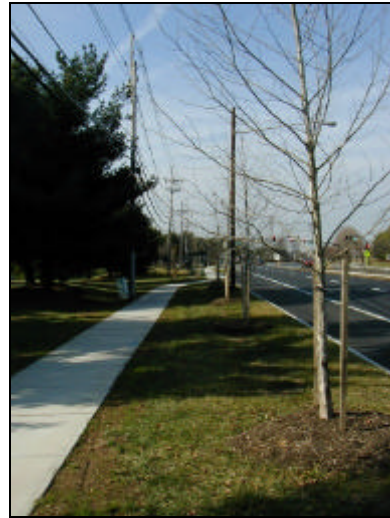
Figure 7: After - Curbs, Sidewalk, Trees
