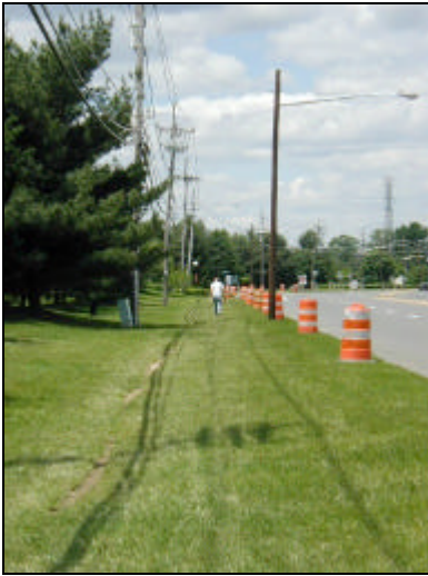
Figure 6: Before - No Curbs, Sidewalk, Or Trees
