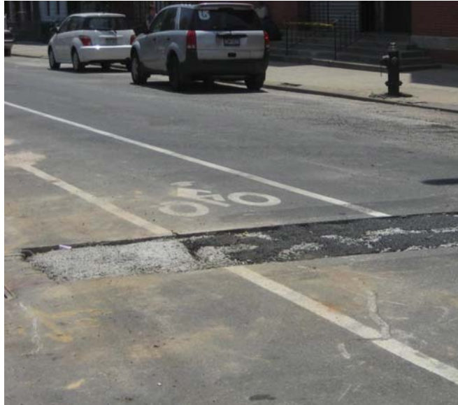
Figure 27: Roadway construction, potholes, utility covers, drain grates and otherwise uneven pavement make cycling on some lanes dangerous.
