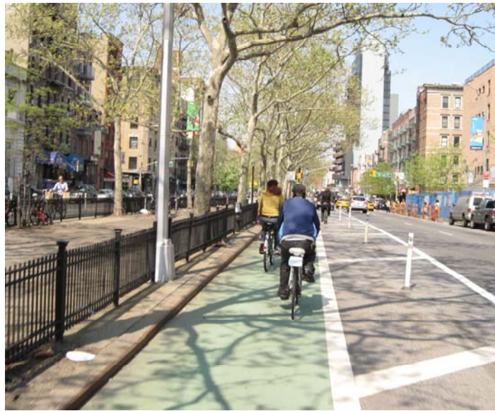
Figure 14: This cycle track along Allen Street in Manhattan provides safe, convenient, and pleasant cycling, completely separated from motor vehicle traffic (Source: Nicholas Klein)
