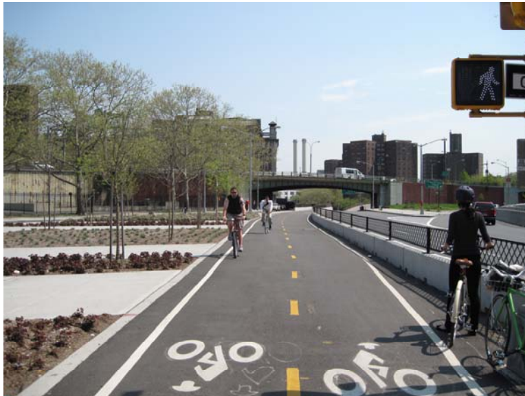
Figure 17: The Sands Street cycle track in Brooklyn, near the Manhattan Bridge, is bi-directional and offers complete separation from motor vehicle traffic. (Source: Nicholas Klein)
