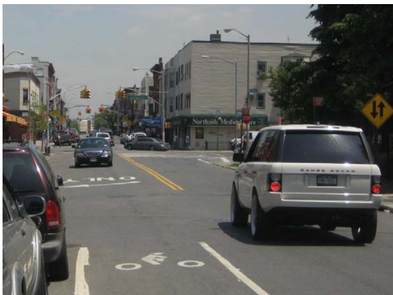
Figure 29: Some bike lanes end abruptly, such as this one in Greenpoint, Brooklyn, forcing cyclists into dangerous conflicts with on-coming motor vehicles.
