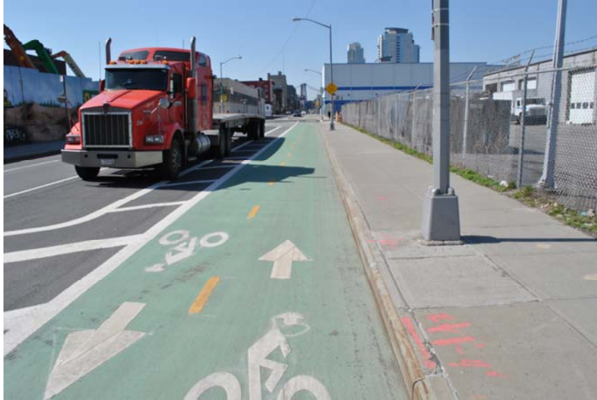
Figure 18: The buffered bi-directional bike lane on Kent Avenue in Williamsburg provides some separation from heavy car and truck traffic on this arterial. (Source: Devin Reitsma)
