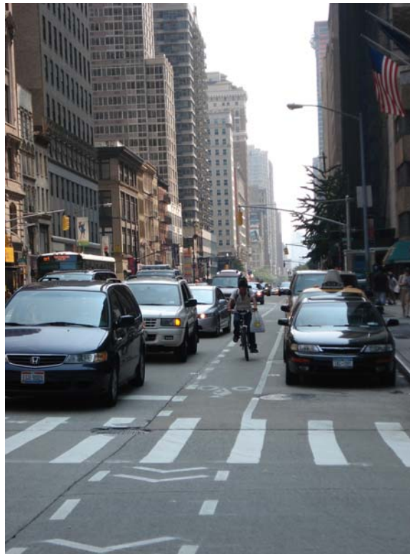
Figure 24: Many bike lanes in New York are too narrow and subject cyclists to the dooring hazard because of the proximity to parked cars, as here on 6 th Avenue in Manhattan. (Source: Ralph Buehler)
