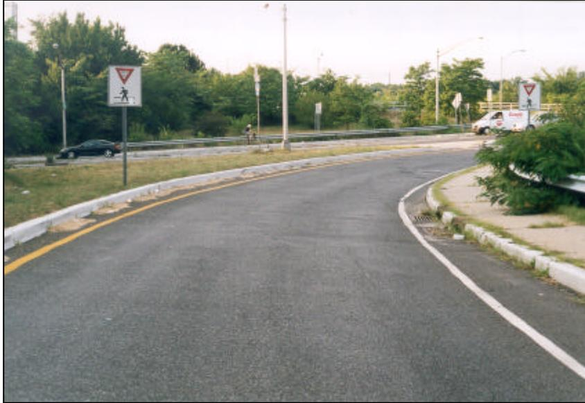
***Picture 3.1-4: Dangerous design and location of crosswalk due to limited sight distance. Although signage alerts motorists of an upcoming crosswalk, it is hidden behind the curve (and bushes). Motorists on this slip lane are looking for gaps to the left. They often turn and even accelerate without noticing pedestrians and cyclists trying to cross. In addition, people crossing cannot see approaching cars. New Brunswick, NJ.***
