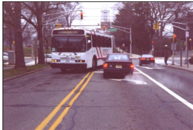
**Picture 3.6-2: Recessed stop line allows bus to turn besides a very tight turning radius – New Brunswick, NJ.**
