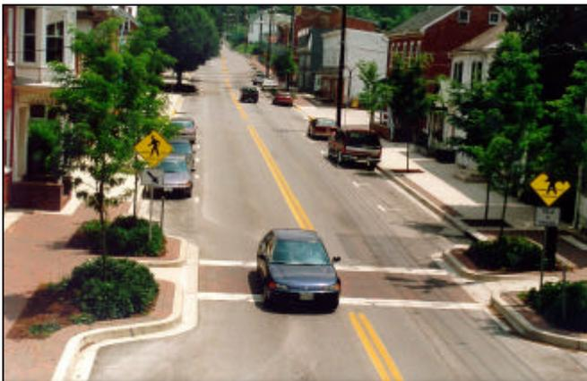
***Picture 3.1-2: Mid-block crossing with curb extension to reduce crossing distance for pedestrians. Westminster, MD.***
