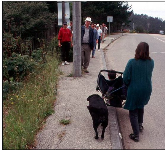
This utility pole blocks the pedestrian zone. (Dan Burden, www.pedbikeimages.org)
