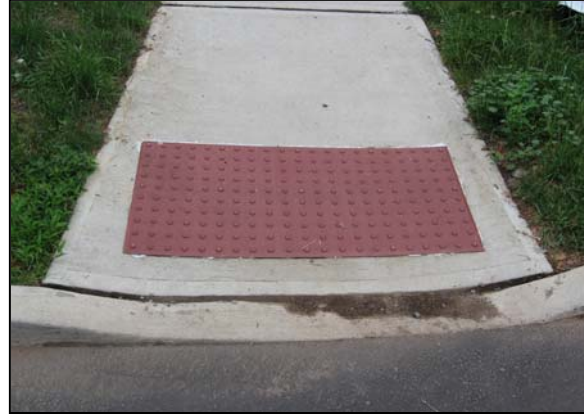
Curb ramp with detectable warning strip, Highland Park, NJ (VTC)
