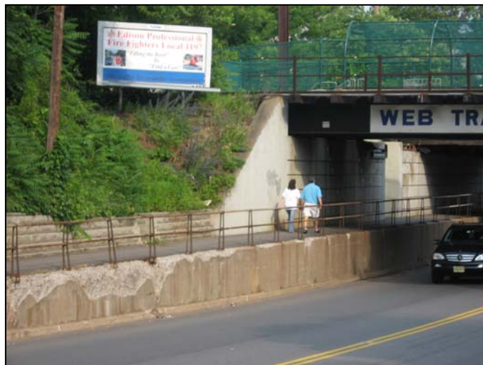
Elevated sidewalk as part of an older underpass of a rail bridge in Edison, NJ (VTC)
