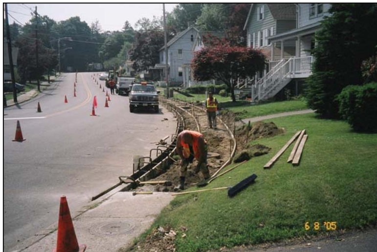
Sidewalk improvements as part of a state highway project in Netcong, NJ (VTC)
