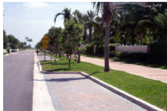
Figure 6.16: Valley Gutter
