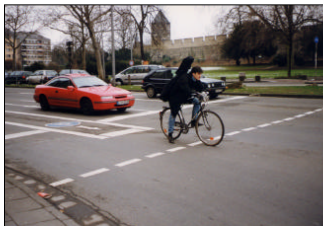
Picture 66: Staggered Stop Lines, Koeln, Germany (MK)
