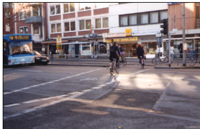
Picture 70: Broken cycle lane through intersection, Germany (MK)
