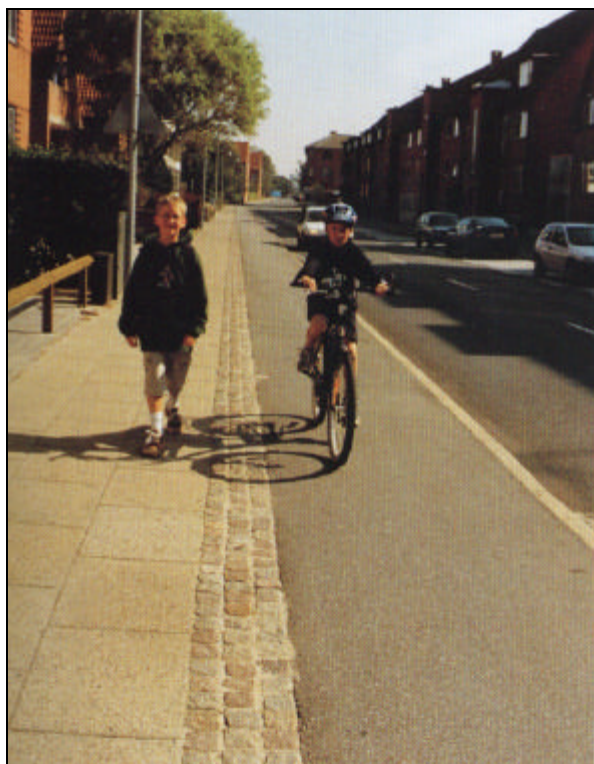
Picture 52: Cycle-Footway with Effective Separation (DK)
