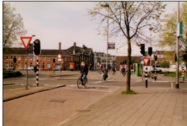
Picture 14: Separate cycle facility at signalized intersection, Germany. (MK)
