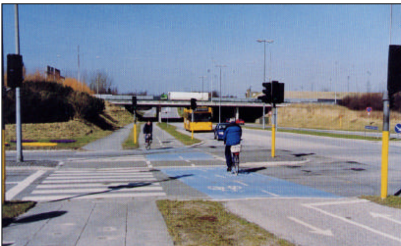
Picture 12: Blue bike lane crossing marked through intersection. (DK)
