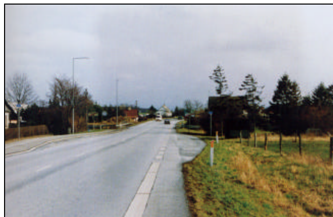
Picture 50: Paved shoulder and Bus Bay (DK)
