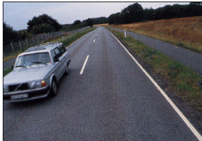
Picture 44: Cycle track with dividing verge, Denmark (DK)
