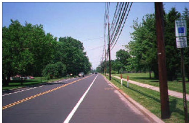
Picture 2: Wide paved shoulder accommodating bicycles. NJ. Source: VTPI.
