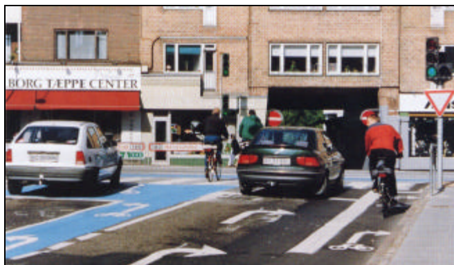
Picture 69: Cycle lane for left-turning cyclists (DK)
