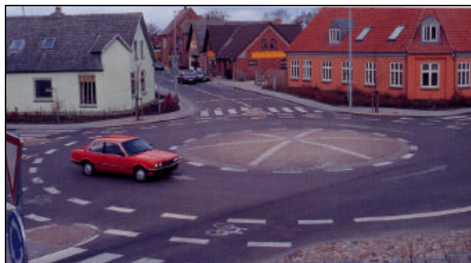
Picture 75: Broken bike lane not ideal since the space is more likely to be used by motor vehicles (DK)
