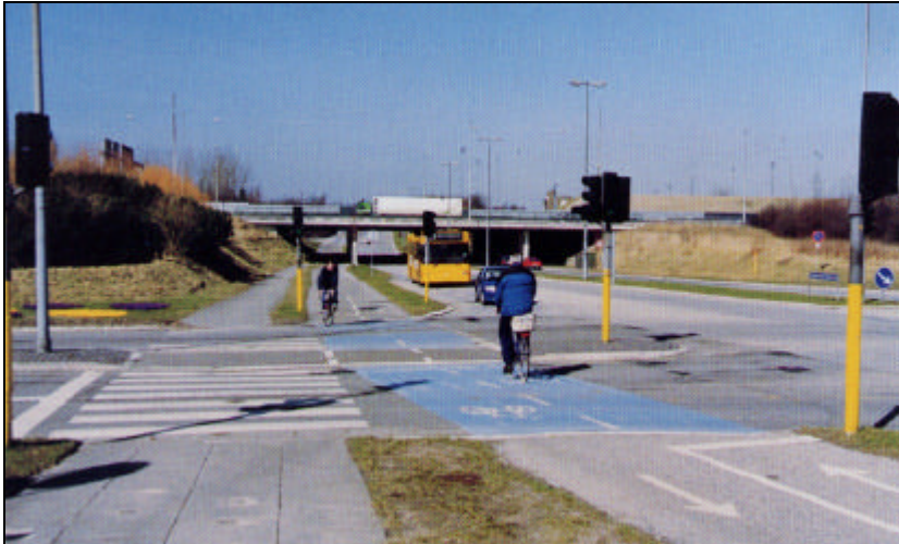
Picture 57: Blue bike lane crossing marked through intersection (DK)
