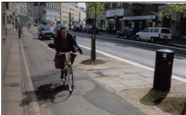
Picture 31: Cycle track in Denmark (MK)
