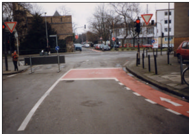
Picture 71: Advanced Stop Box, Koeln, Germany (MK)
