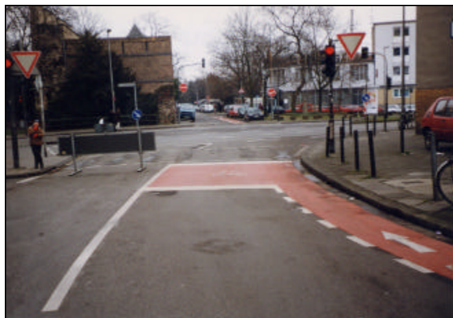
Picture 25: Advanced Stop Box, Koeln, Germany. (MK)
