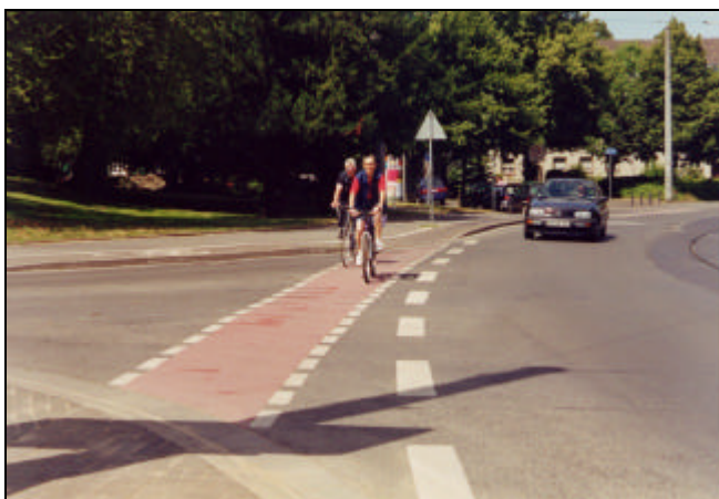
Picture 55: Cycle track continued as colored lane through intersection (MK)
