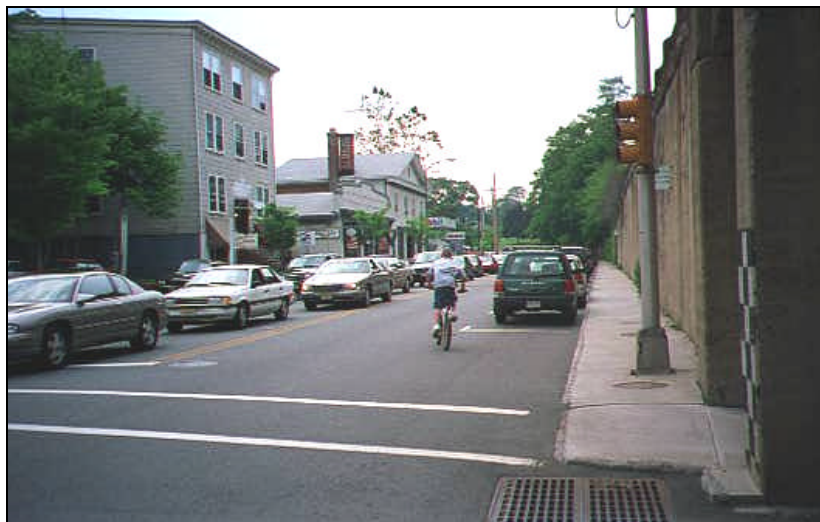
Picture 10: Limited space to provide bike lane, wide outside lane or shoulder leaves the options to either eliminate parking or to introduce a speed limit of 20mph or less to allow cyclists to safely take the lane. (MK)
