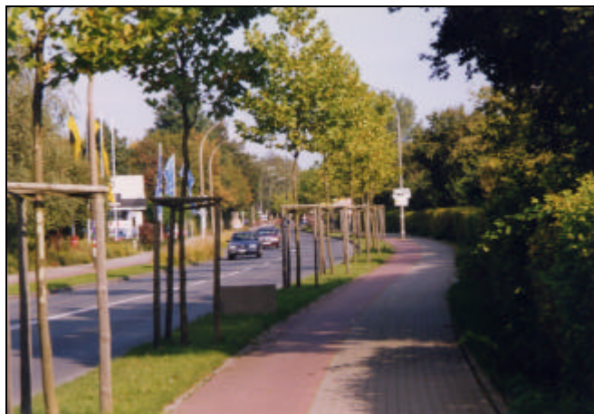
Picture 43: Cycle track with dividing verge, Germany (MK)
