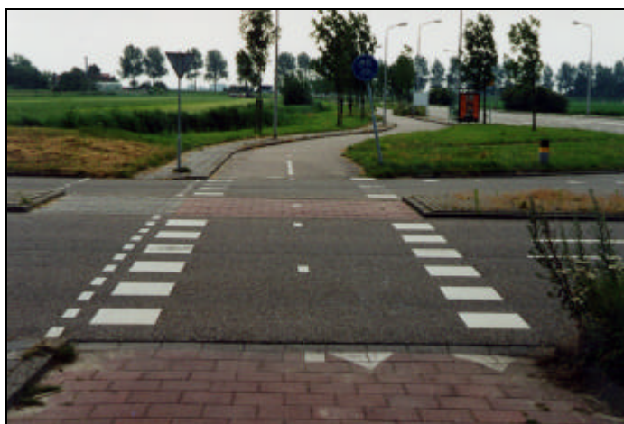
Picture 17: Bend-out cycle track (suburb of Amsterdam). (PS)
