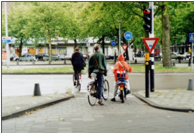
Picture 58: Separate cycle facility at signalized intersection, The Netherlands (PS)
