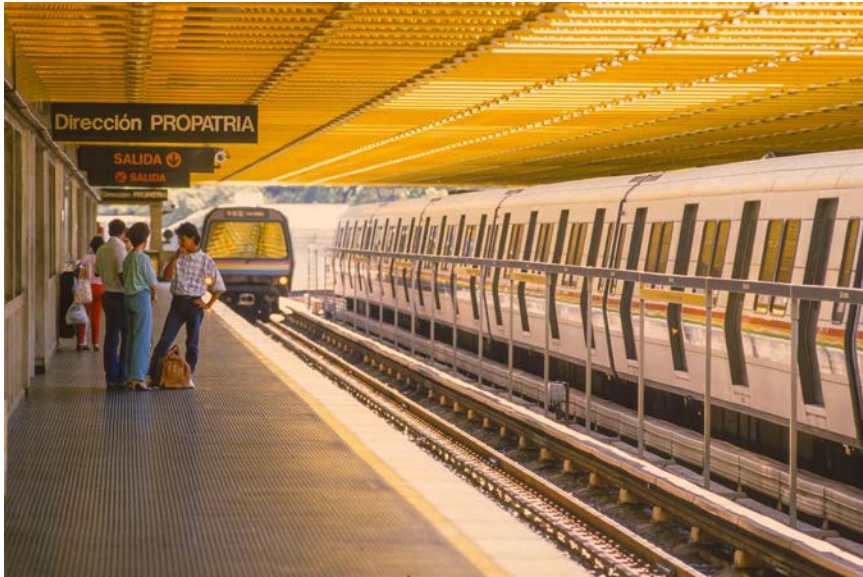
AMV's estimate of peak demand helped determine the necessary length of trains and operating frequency for the Caracas system. Image: Rob Crandall / Alamy
