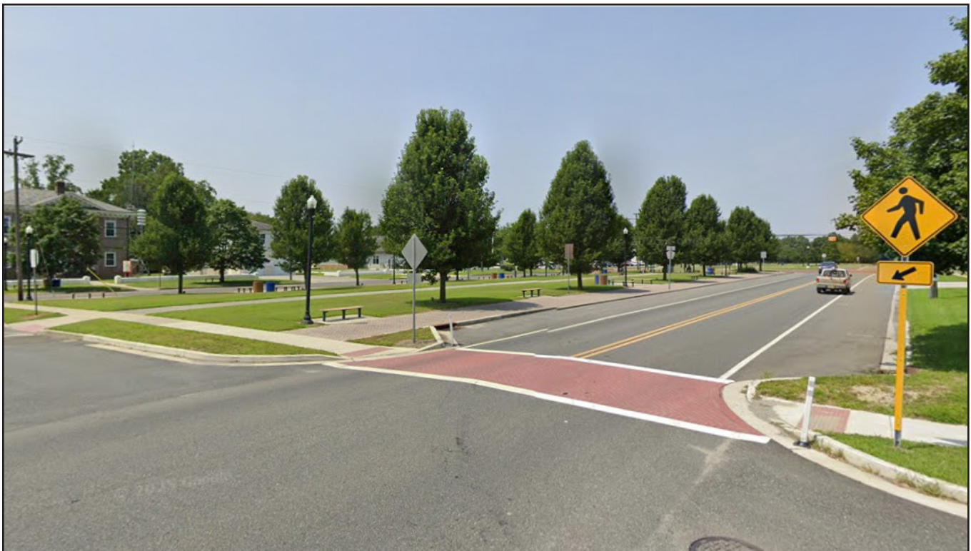
Figure 21. Concrete Curb Extension Near Intersection in Woodbine, NJ (Google StreetView)
