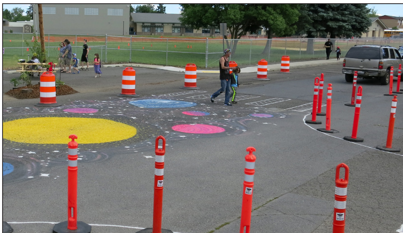
Figure 22. Example of a Temporary School Zone Crosswalk, Street Mural, and Curb Extension (National Complete Streets Coalition)
